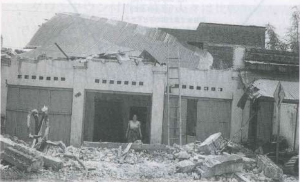
Damage by Earthquake at Pinrang
