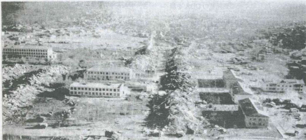
Debris of collapsed structures due to the 1995 Sakhalin earthquake (Courtesy of Dr. J. M. Eisenberg, Russian National Delegate to IAEE)
